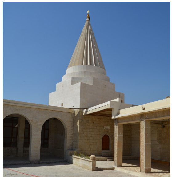
Figure 29b: The shrine of Pir Bob post-reconstruction, April 2018 (©Faris Mishko/Used With Permission)
