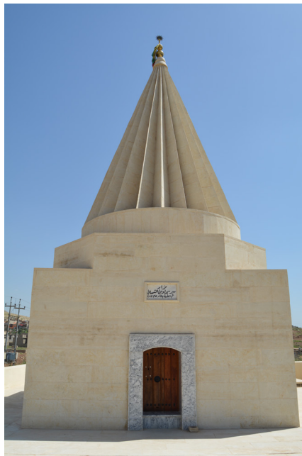
Figure 31a: The shrine of Mer Sjadeen post-reconstruction, April 2018 (©Faris Mishko/Used With Permission)
