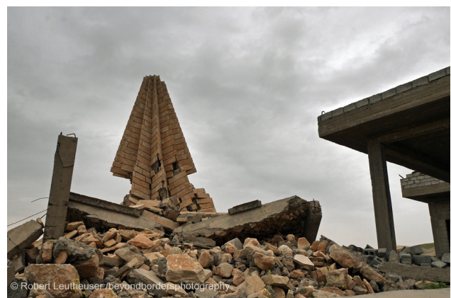
Figure 13b: The shrine of Sheikh Hassan post-destruction, April 2017 (©Robert Leutheuser/All Rights Reserved)
